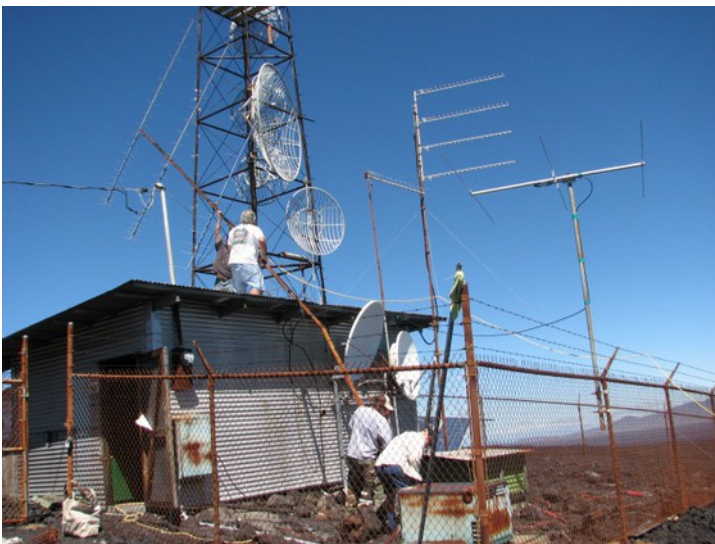
Repeater Shack Facing West
