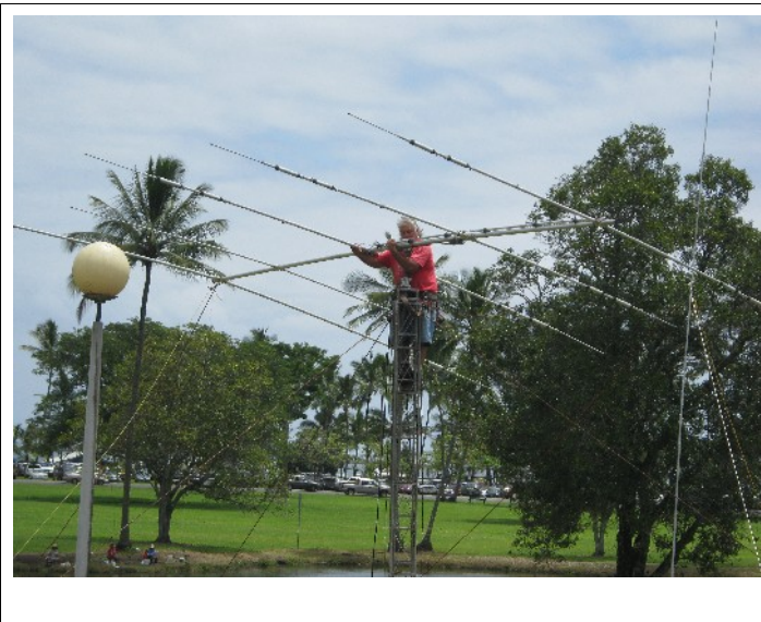
Milt AH6I's Yagi on its way up
