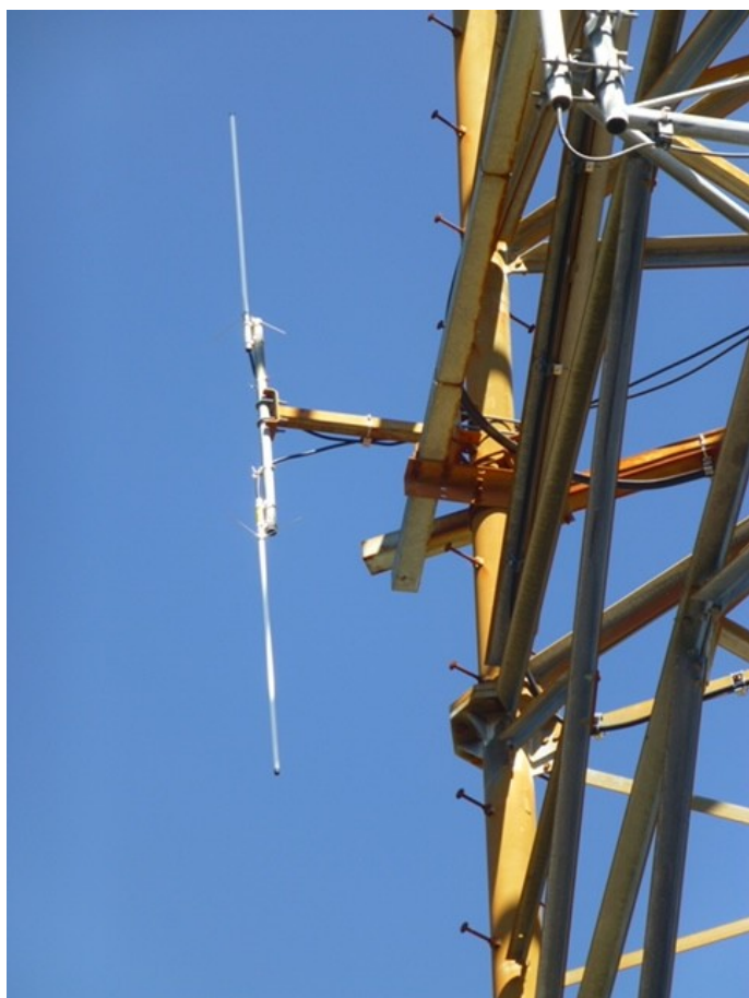
The new BIARC antennas, mounted in a closely spaced Siamese arrangement.
