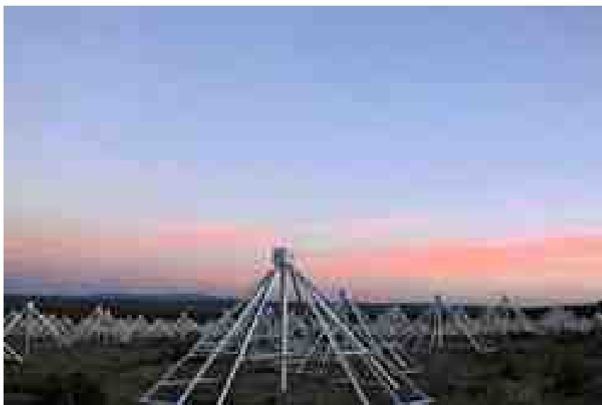
The Long Wavelength Array at Sevilleta National Wildlife Refuge is capable of imaging the entire sky at once, allowing AFRL scientists to track and characterize sporadic E. The facility consists of 256 dual-polarization dipoles.
